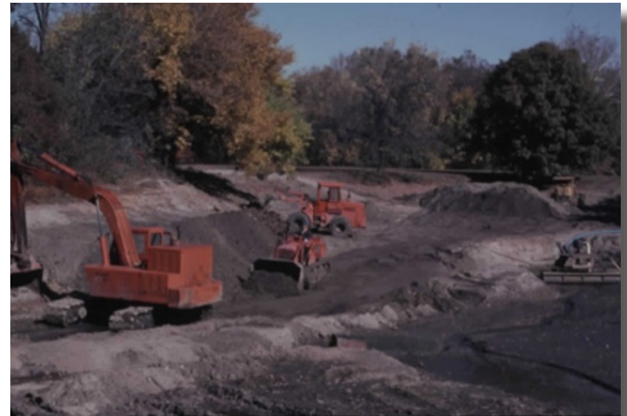
The excavation and rehabilitation of 1985
